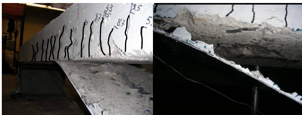
Figure 4.2 – Debonding failure exhibited by the specimen EB
